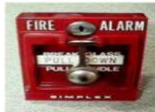
Fire alarm pull stations
